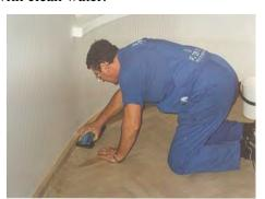
2) paint or other building products dropped onto the wood surface can be removed by scraping with something as fine as a Stanley knife blade.
