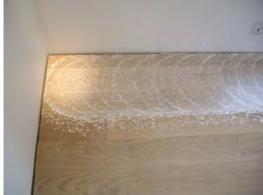
This is a nice even application of oil. Where necessary, apply up to room edges by hand. Allow the oil 30 minutes to absorb and during this period buff it into the wood using an olive nylon pad under your
