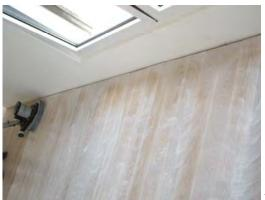
Buff the floor twice with a nylon pad under which is placed 2 orange, fine grade patina disks. This is optional – whilst Patina disks give a smoother feel to the floor they can strip an amount of colour from the wood surface – its important to test the process in advance. An alternative is to oil without patina disks to get a particular colour then allow smoothness to come through time and cleaning.
