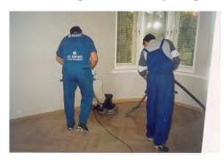
Cleaner from the polisher's tank. If there is no tank then apply using a sponge. Work over the floor allowing the weight of the machine to evenly clean the floor.
