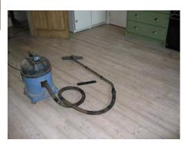
If this equipment is not available then use the Doodlebug with Scrub Pad to mop the surface. Continue to rinse the mop as you proceed since the objective is to remove excess Lye solution.
