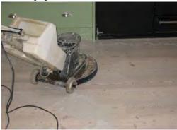
5) Before moving onto Stage 2 ensure the floor is thoroughly dry: 8 hours at 20 deg,C or overnight, in other words.
